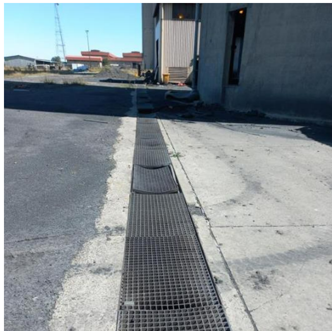
Figure 22: Concrete Drains Surrounding Each Coal Silo
