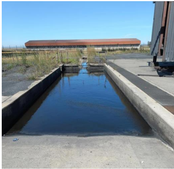
Figure 23: Silt Trap at Each Silo
