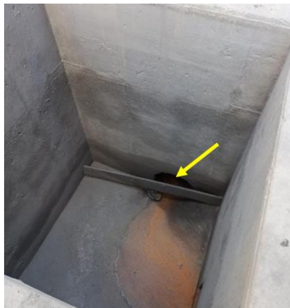
Figure 5: Outlet Pipe to Station Drains
